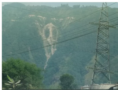
Land slide due to non-engineered hill road
