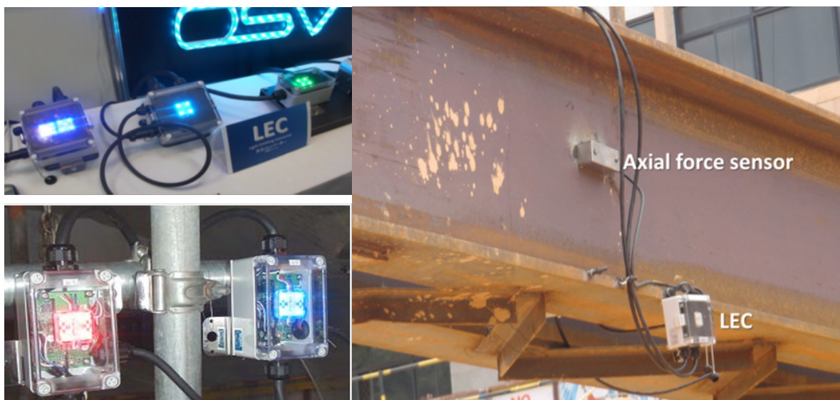
Fig. 6 Using LEC at excavation site (M.NOMURA, 2015)
