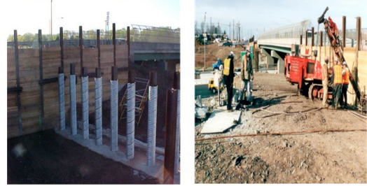
Pile with Cushion Tie Back Wall
