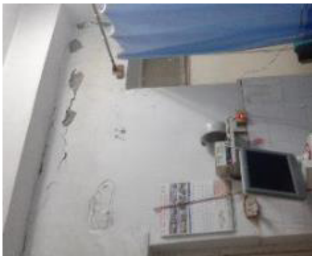
Photos 1: Damages due to Gorkha Earthquake in CT Scan & ENT Blocks
