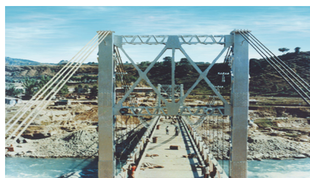
Trishuli Suspension Bridge at Nepal
