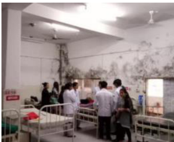
Photos: Serious seepage issues inside Emergency Block & Corrosion Cracks in the structure members
