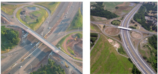
I-95 Road Bridge-Progress Br. Completed
