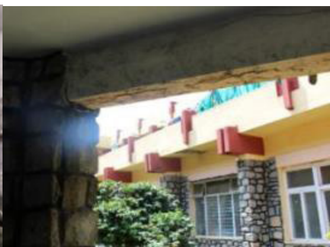
Photos: Serious seepage issues inside Emergency Block & Corrosion Cracks in the structure members
