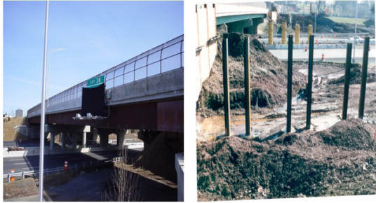
I-95 Scotch Road (Integral Abutment Design)
